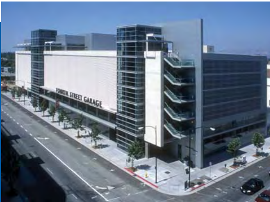
Fourth Street Garage
