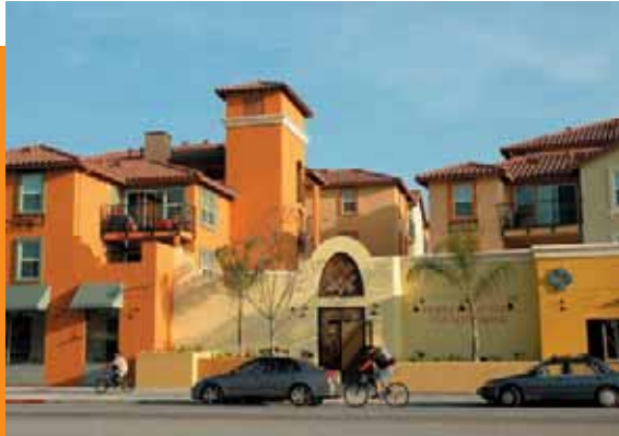
Tierra Encantada Affordable Housing
