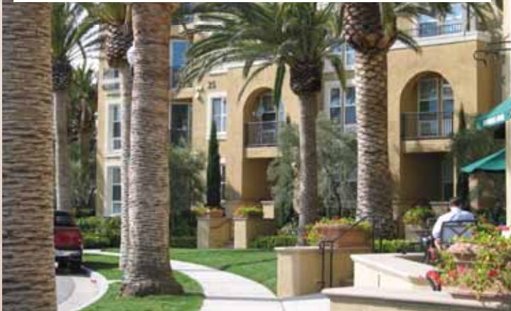
Typical Elevated Residential Building
